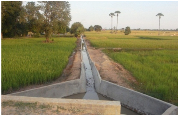
Figure 10: Concrete canal receiving water from the reservoir to irrigate nearby rice fields during the dry season December 2012
