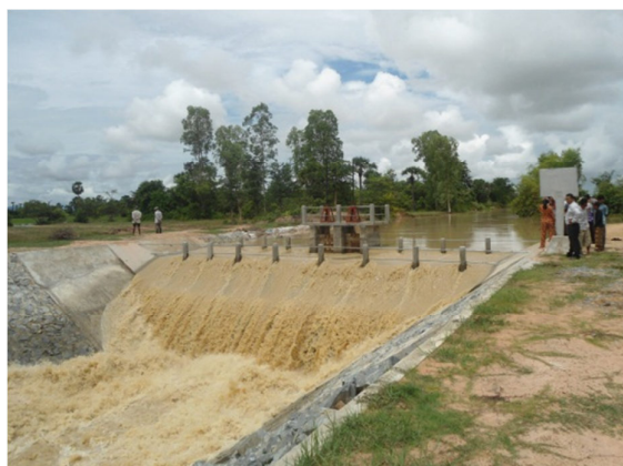
Figure 7: Spillway finally constructed to keep the water for irrigation in the target area
