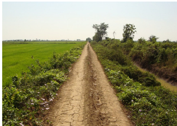
Figure 7: Restored canal embankment to work as a road and dike
