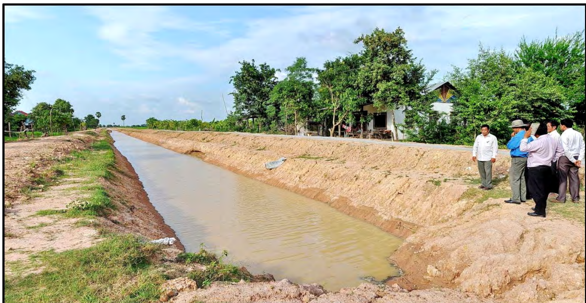
Figure 4: Canal Under Rehabilitation (Tnaot Commune)
