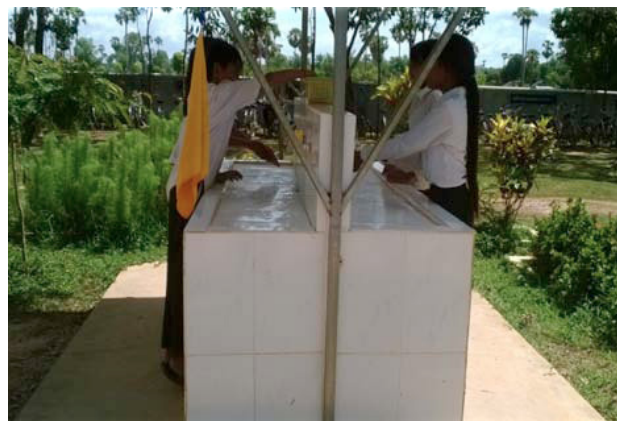
Innovations in WASH Design: New Hand Washing Station that allows access to multiple students at the same time.
