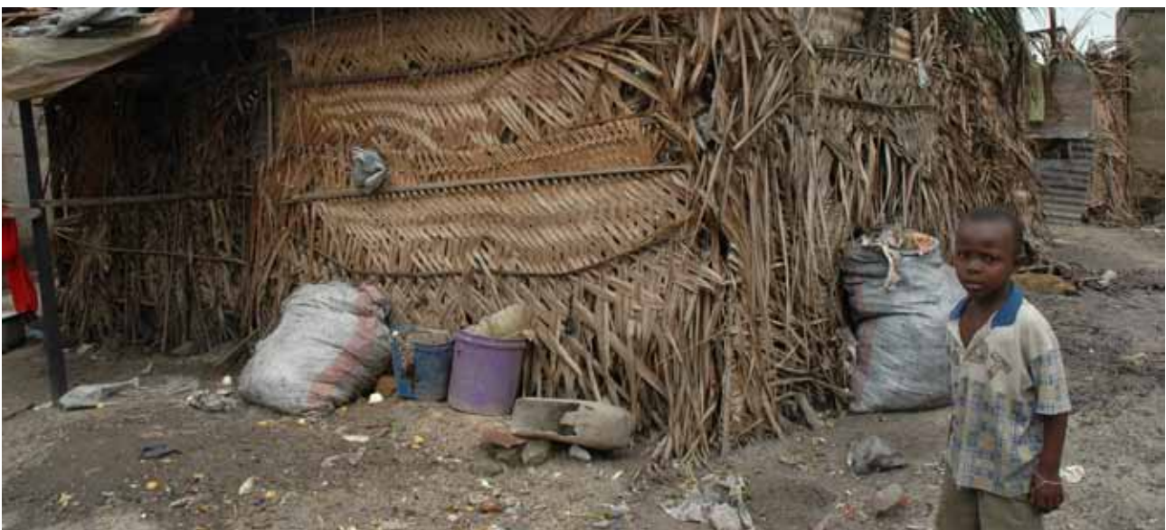
Fragile structures in Manzese, a densely populated neighbourhood in Dar Es Salaam, Tanzania. © UN-Habitat/Suzi Mutter
