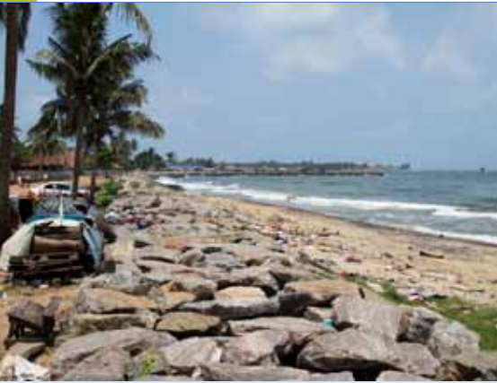
Negombo seawall. © UN-Habitat/Bernhard Barth
