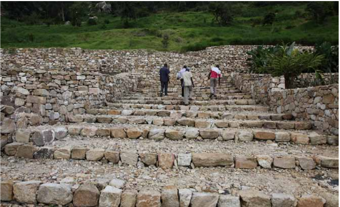
Reclaimed disaster prone hills as a park after relocation of residents to a safer place in Rubavu, Rwanda.
