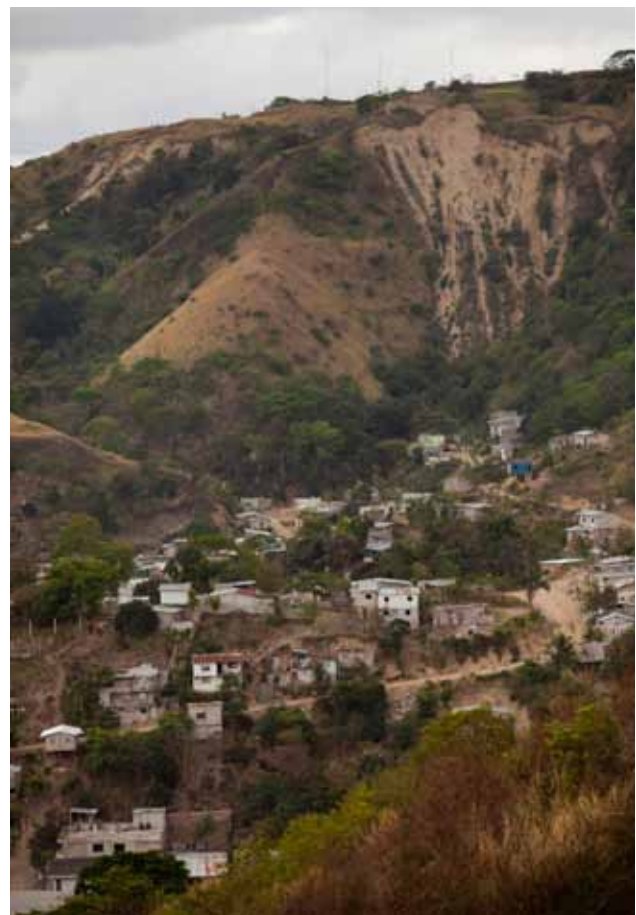
A landslide in Cerro del Barrio Lindo gatazo affects several houses built on hillsides in Esmeraldas, Ecuador.
