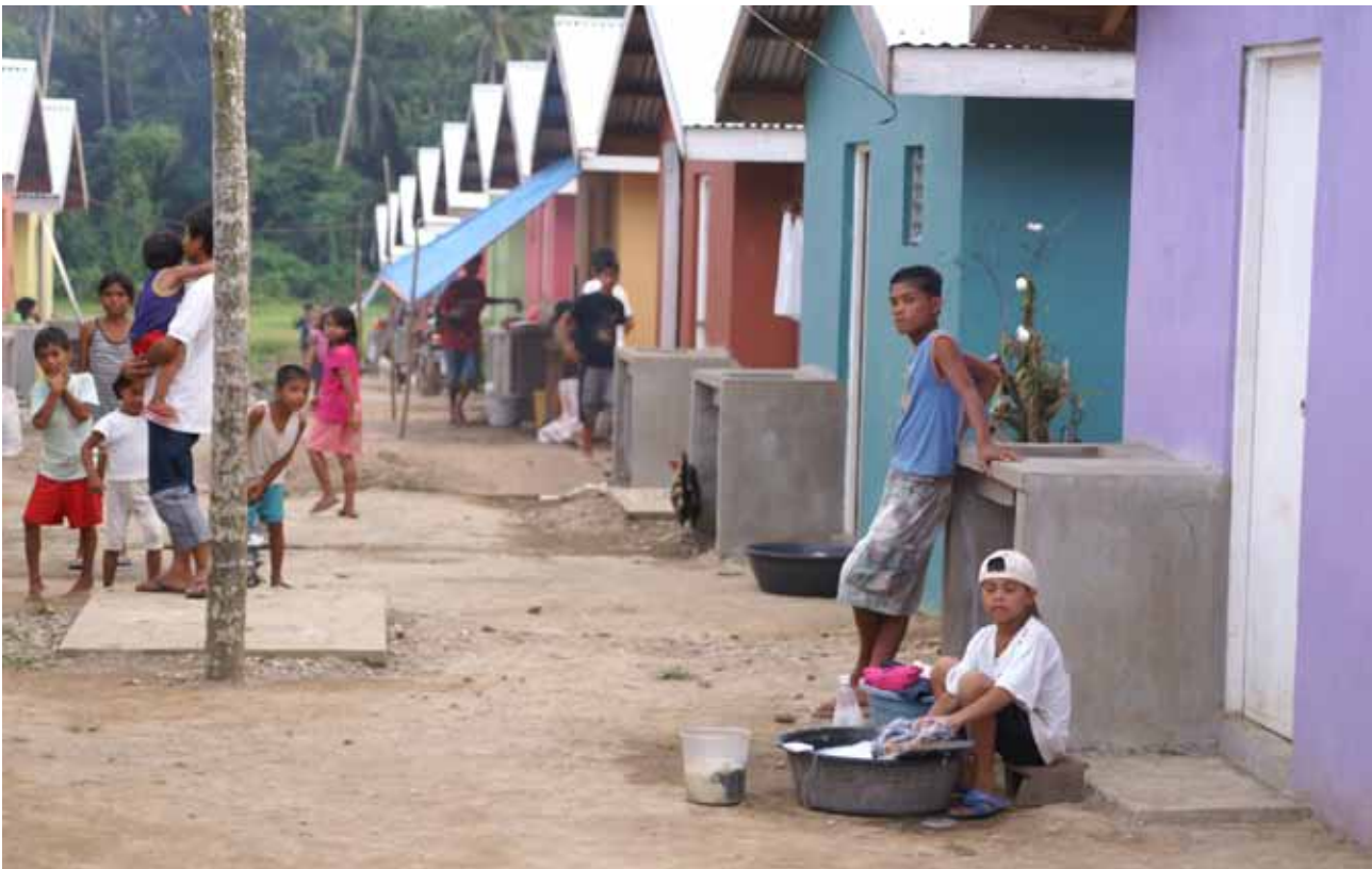
Housing programme accommodating displaced coastal communities, Philippines. © UN-Habitat/Bernhard Barth
