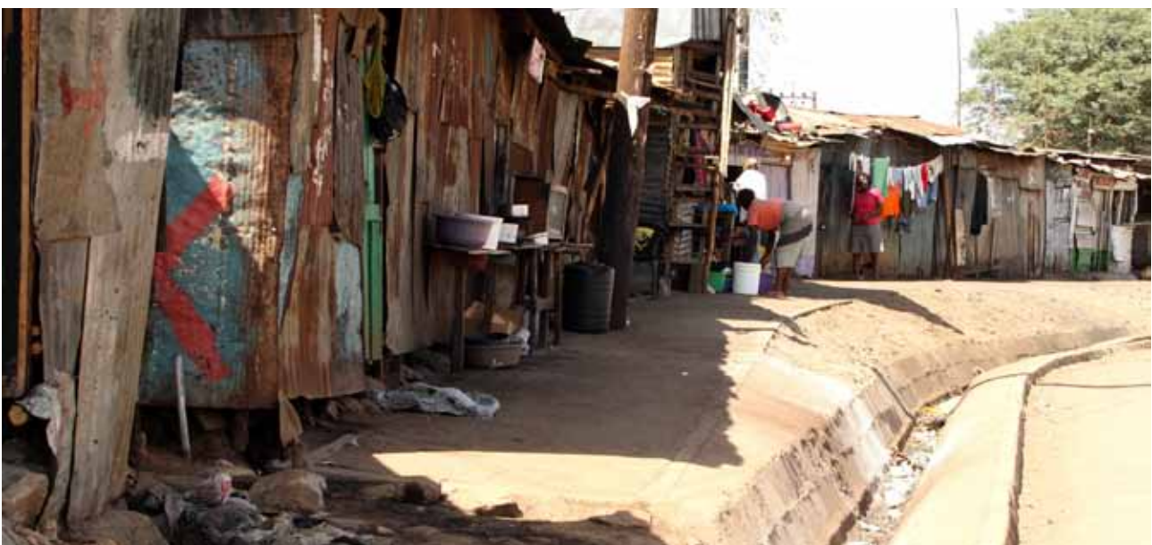
Newly constructed drainage, Kibera. © UN-Habitat/Bernhard Barth
