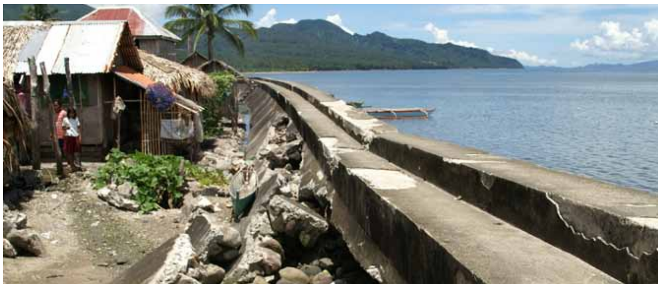
Seawall in Sorsogon City, Philippines © UN-Habitat/Bernhard Barth
