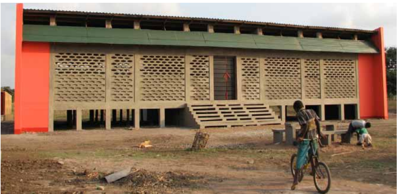
Flood-proof elevated school in Maniquenique, Mozambique. © UN-Habitat/Arianna Francioni
