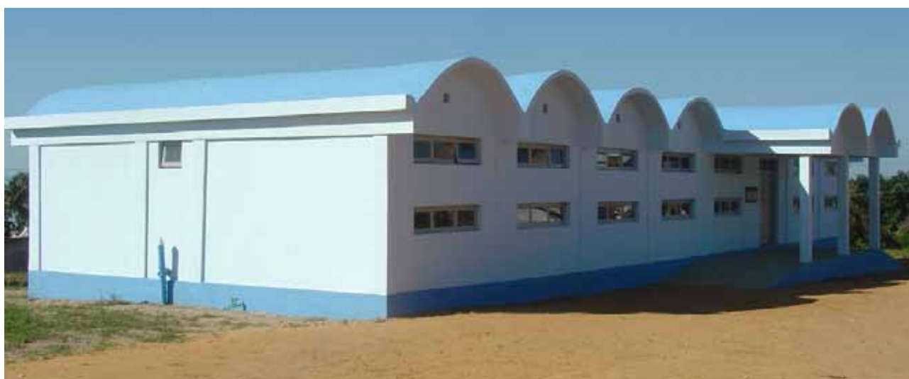
Cyclone-proof kindergarten in Vilankulo, Mozambique. © UN-Habitat/Arianna Francioni
