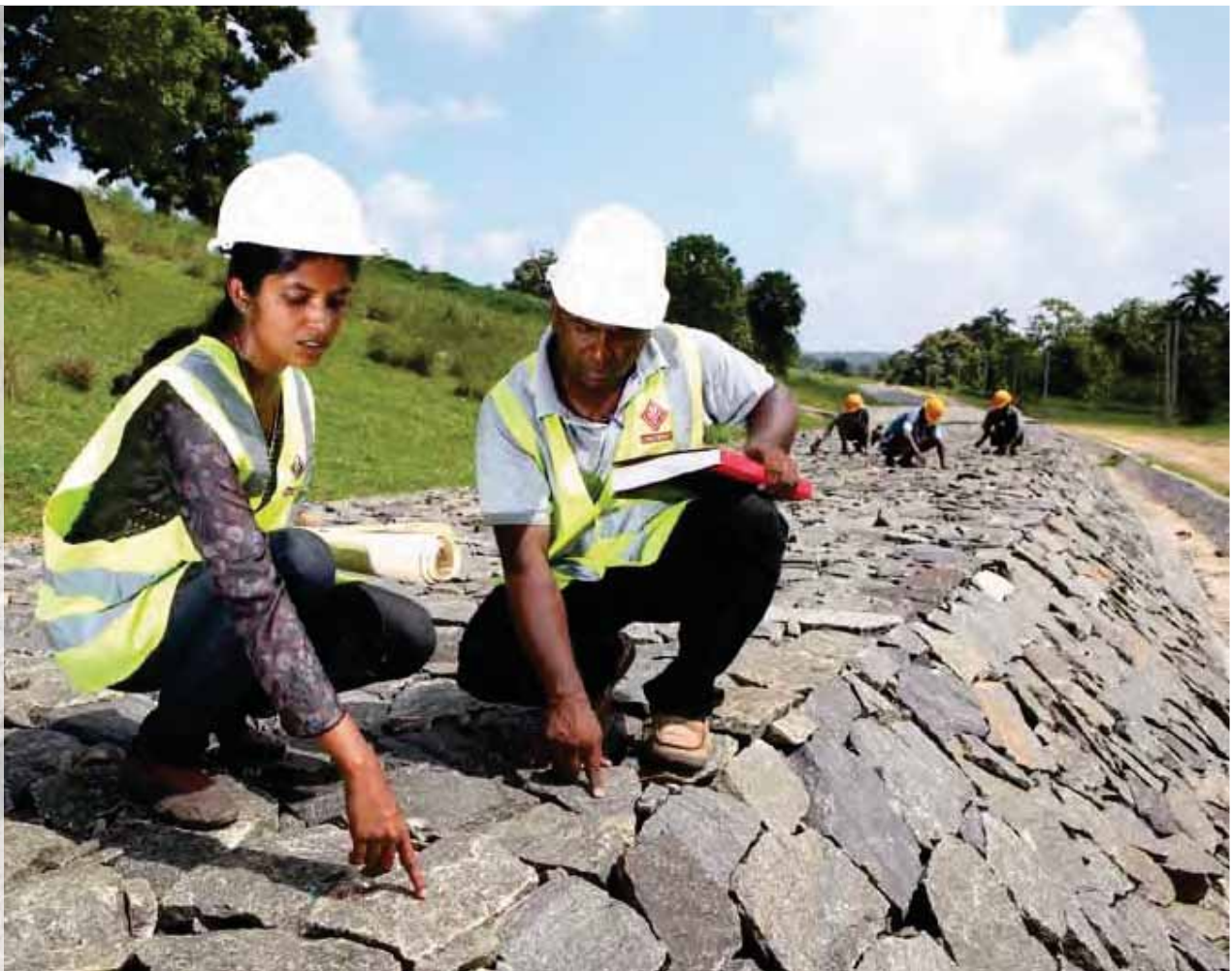
Dam under construction in Sri Lanka. © Lakshman Nadaraja/World Bank
