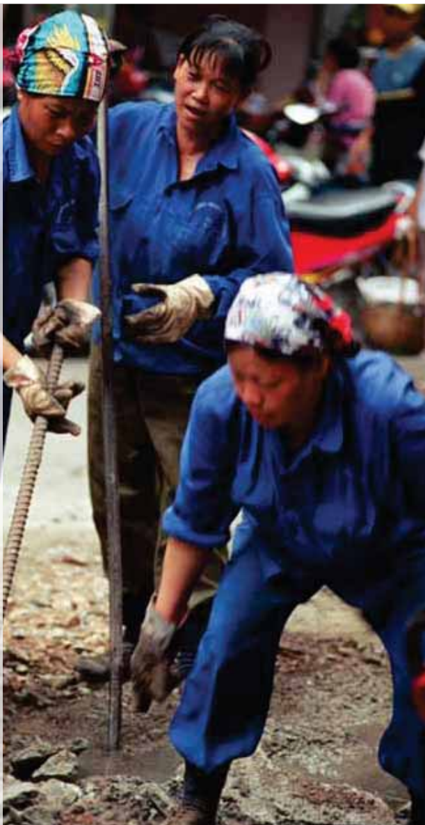
Women repairing a road in Hanoi. ©Tran Thi Hoa/World Bank
