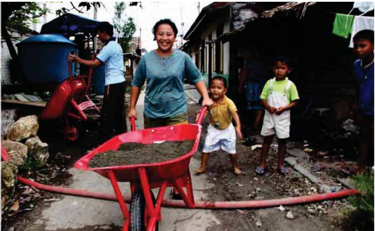
Settlement reconstruction in Nias, Indonesia. 2005. ©UN-Habitat/Veronica Wijaya
