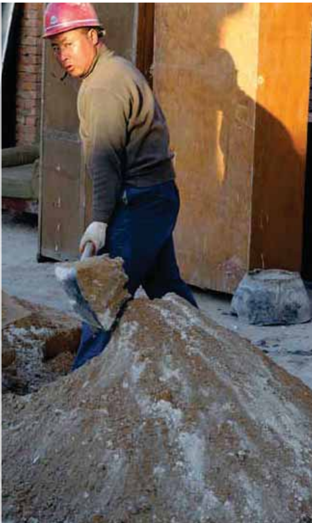
Construction worker at work, Tianjin, China.
