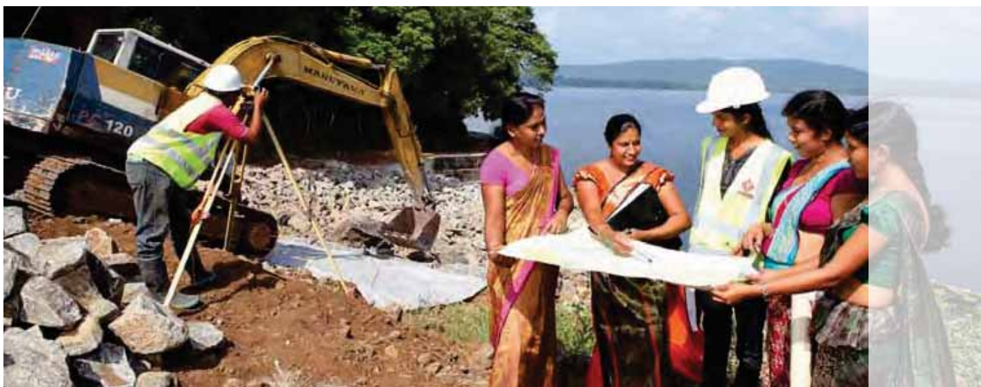
Dam under construction in Sri Lanka. ©Lakshman Nadaraja/World Bank
