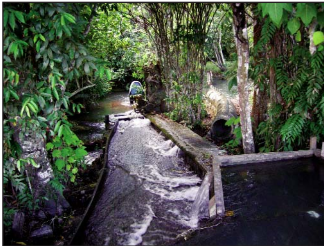
A Micro-Hydropower Project in O Pong Moun, Stung Treng.
