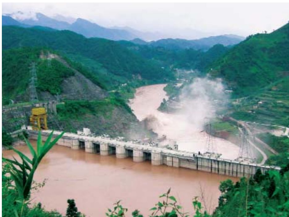
The Manwan Hydropower Dam on the Mekong River in China.
