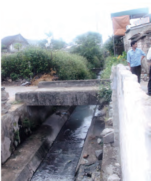
Picture 2. Sharing system of Sewage and drainage in Ben Thuy Ward-Vinh City
