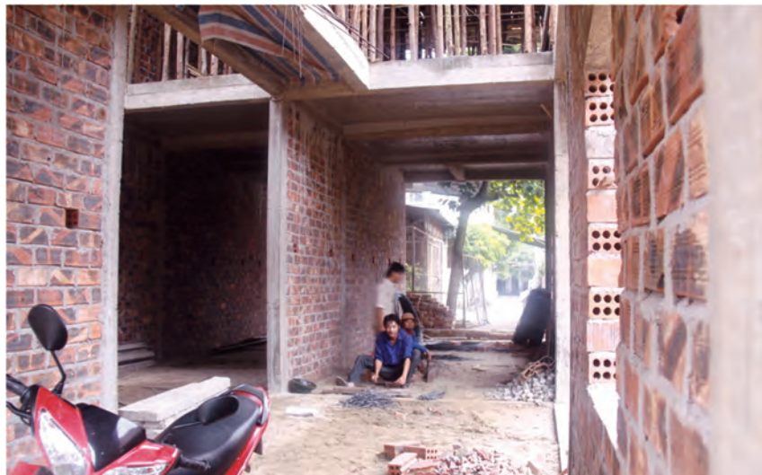
Picture 23. The new houses sharing the wall and foundation being constructed
