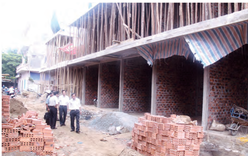
Picture 17. The new houses for households sharing the wall and foundation in the implementation process
