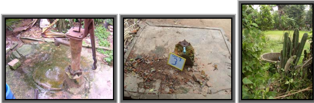
Hole and pump wells found in disrepair and supplying dangerously polluted water to villagers
