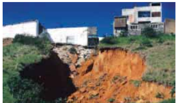
Soil erosion, Maputo © UN-Habitat/Jesper Milner
