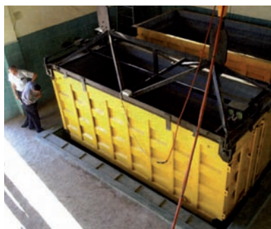
e) Container being lowered into pit
