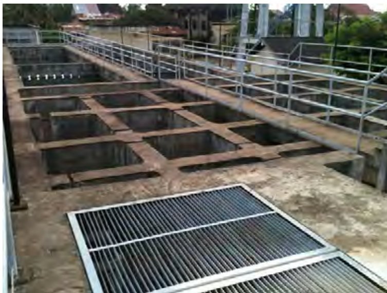
Photo 4.7.1 Flocculator and Sedimentation Basin
