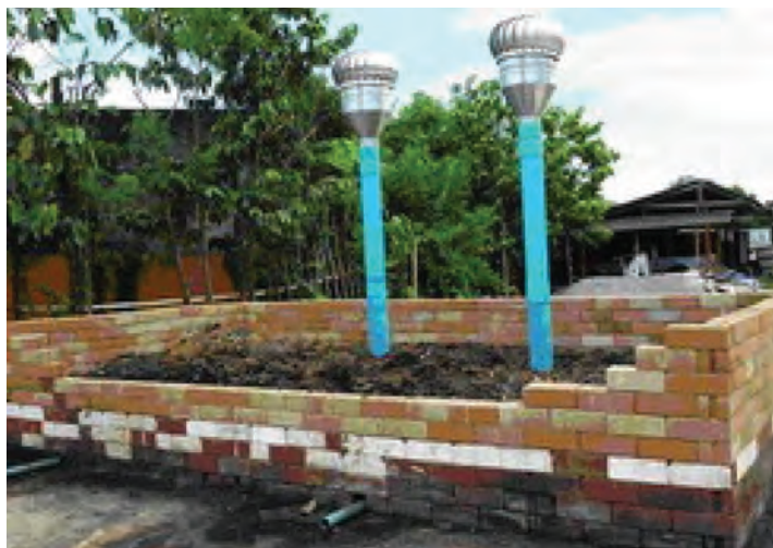
Picture 22. A compost production pit with ventilator and drainage ducts
