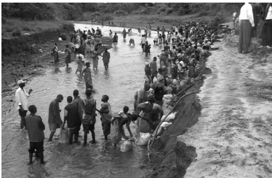
Villagers from Pende village reinforce dyke with sand bags
