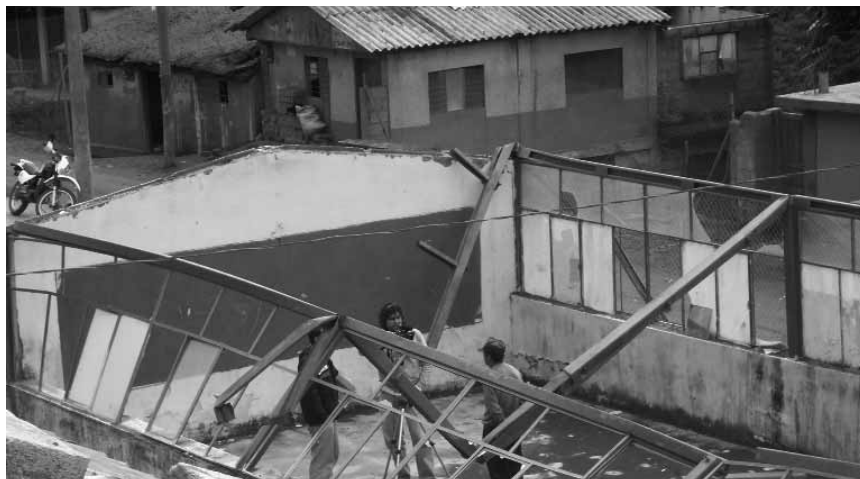
A school roof collapsed under the weight of volcanic ash
